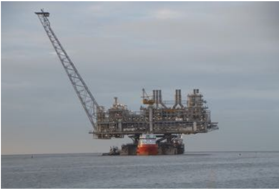
Towing out the new construction Azeri platform offshore Baku.
