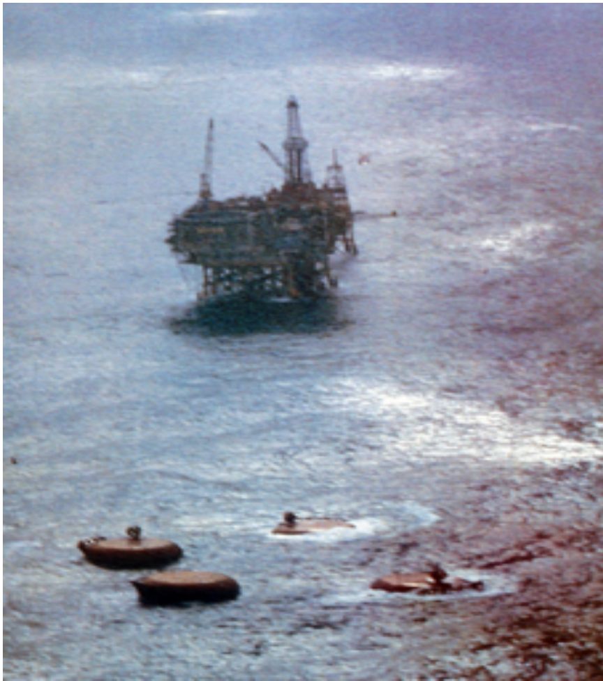
The Alexander Kielland tragedy; the fifth leg is missing.
