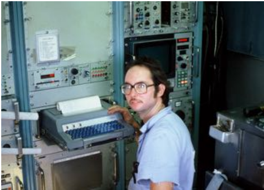
Running the CSU (Cyber Service Unit) on the Ron Tappmeyer . Note the clean-shaven face to be able to wear SCBA emergency air-supply equipment.
